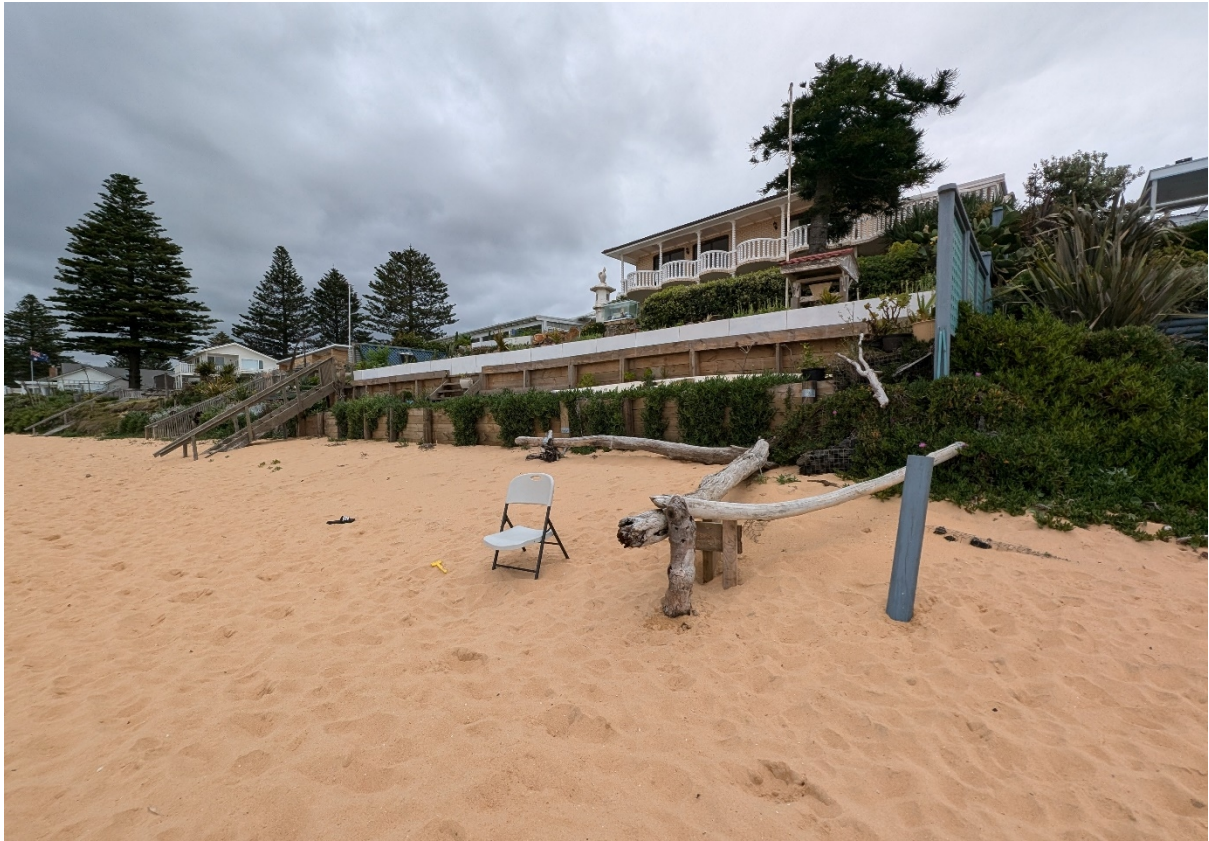
Figure 4 – Ad-hoc coastal protection works
