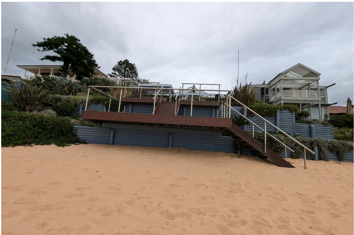
Figure 5 – Ad-hoc coastal protection works
