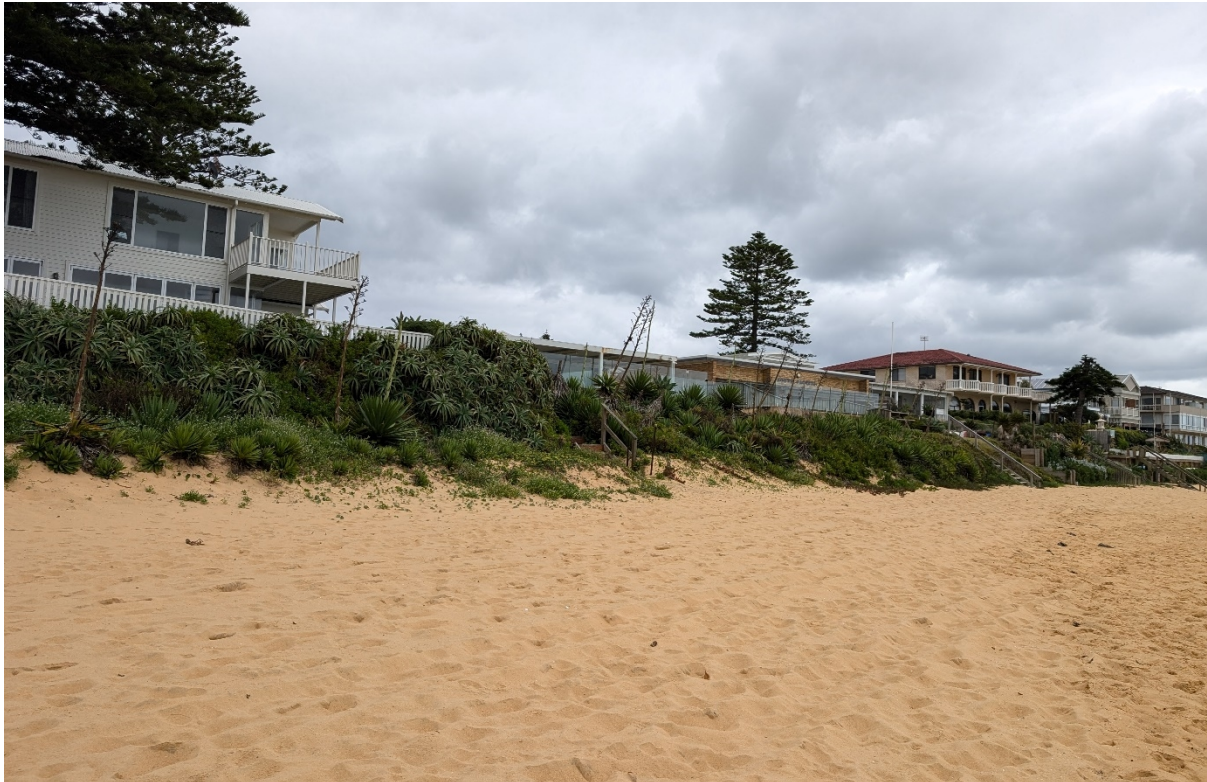
Figure 6 – Ad-hoc protection works and rock placement
